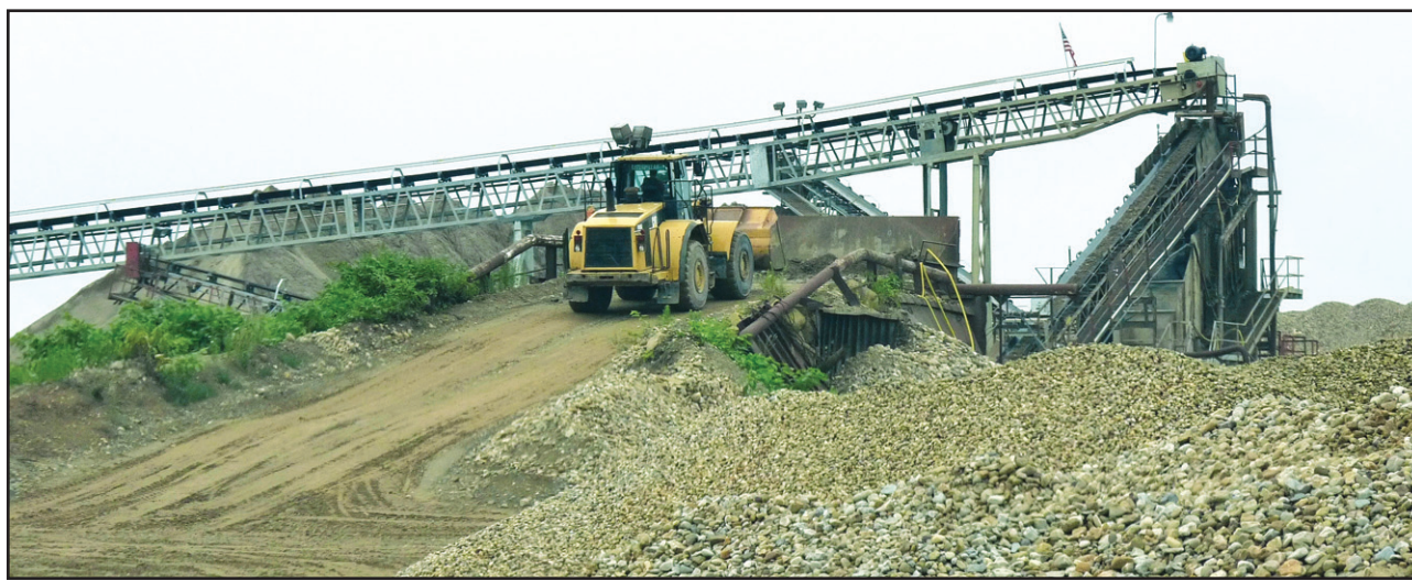
A loader dumps gravel into the primary crusher.
