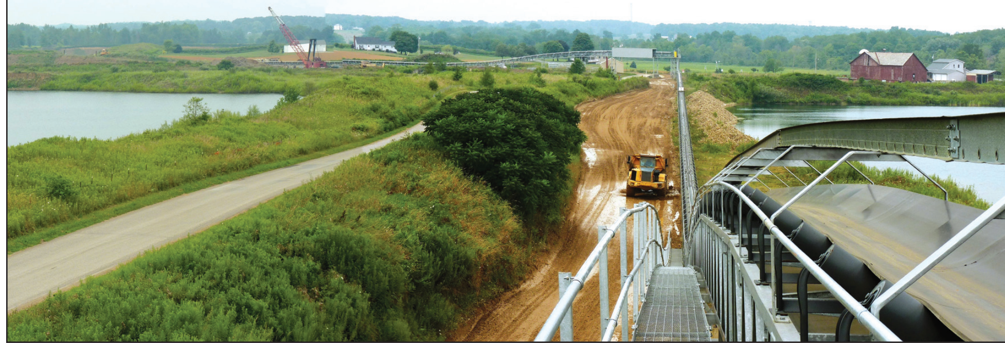
A haul truck brings material to the processing plant while the overland conveyor is in its final days of installation. The dragline crane that mines the sand and gravel is located to the left of the conveyor on the left of this photo.
